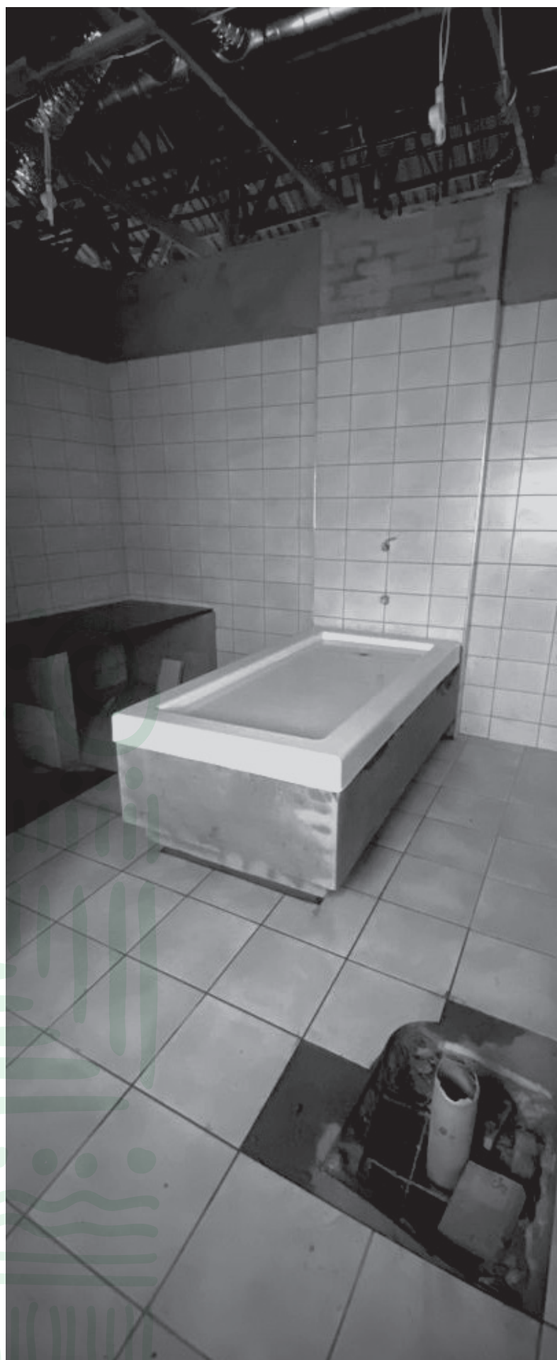
ShowerBath installation process at ERV
